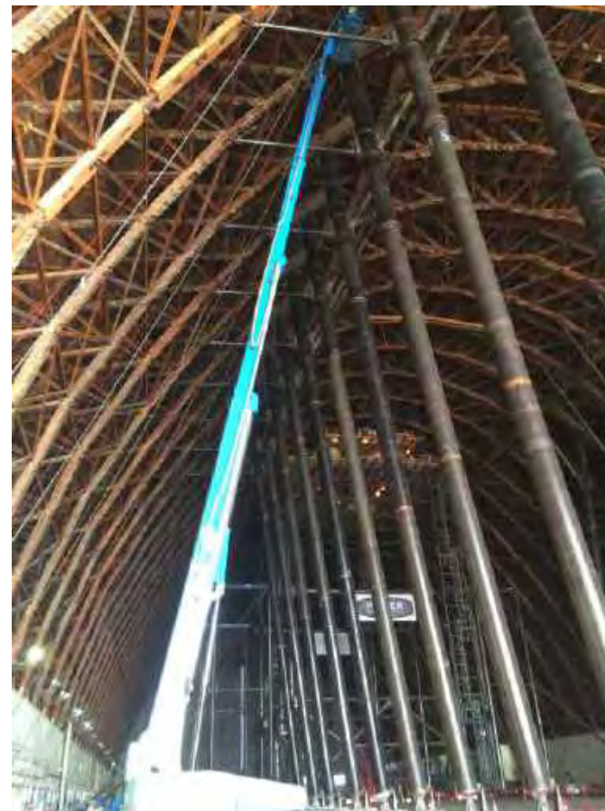
Boom lift used for visual observations
