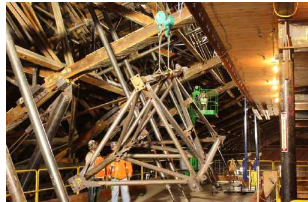
Hoisting exoskeleton segment into place
