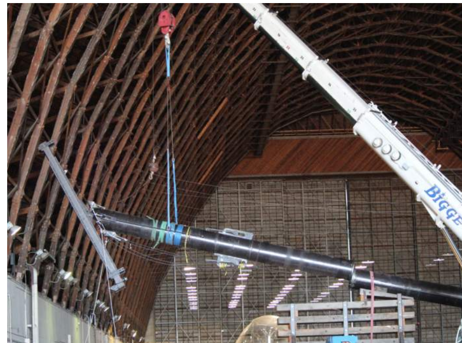
Hoisting of temporary shore segment
