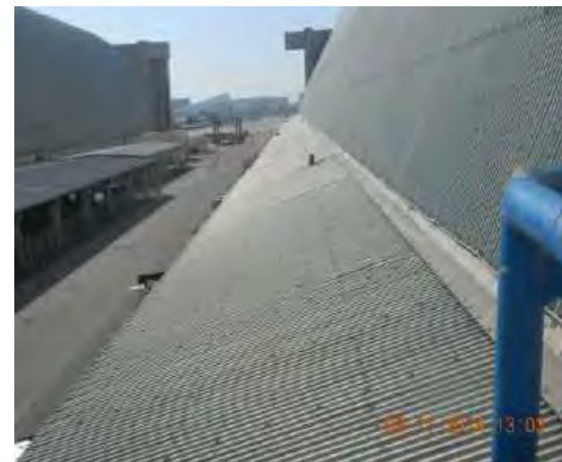
Current aluminum roofing
