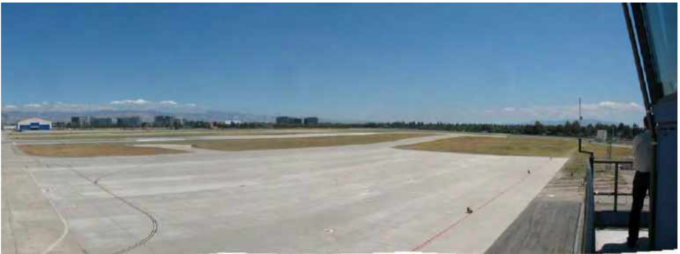
Panoramas of the Airfield. Looking north and northeast toward Hangars 1, 2, and 3 (top); looking east toward CANG and south toward the end of the runways (bottom) (Source: AECOM 2013)
