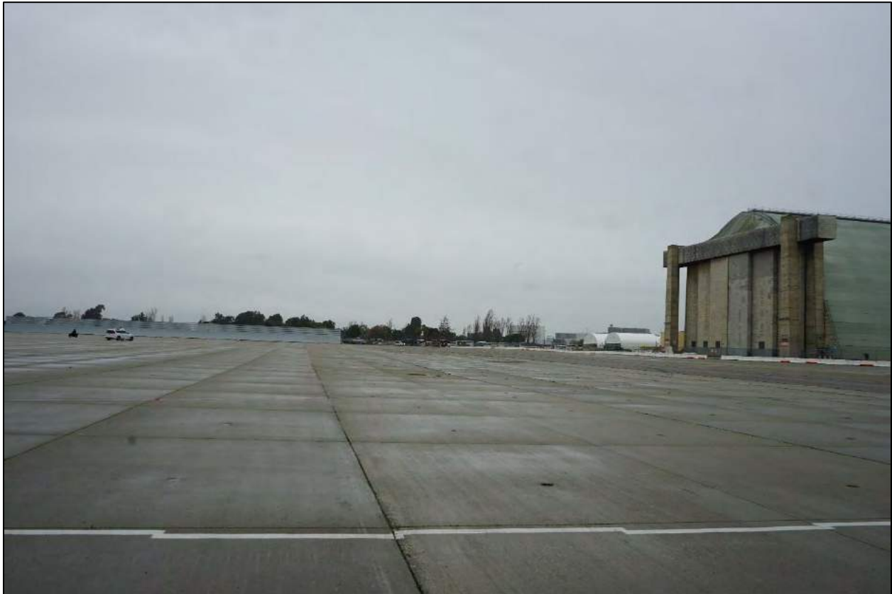
Photograph 6: North portion of East MF1002 exhibiting typical conditions; note Hangar 3 north façade at right.
