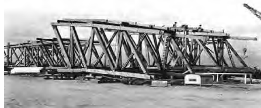
Pre-assembled truss panels awaiting erection -US Navy Historic Photos
