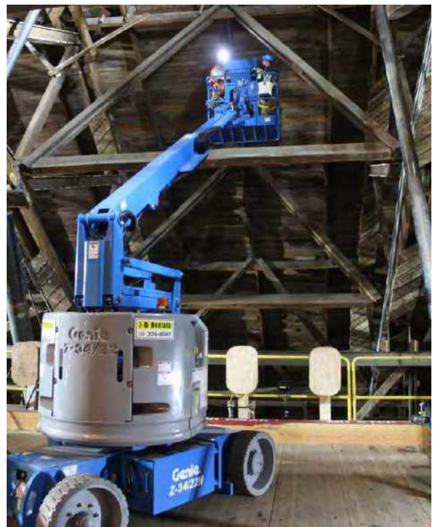
Truss observations from a boom lift on top of access tower
