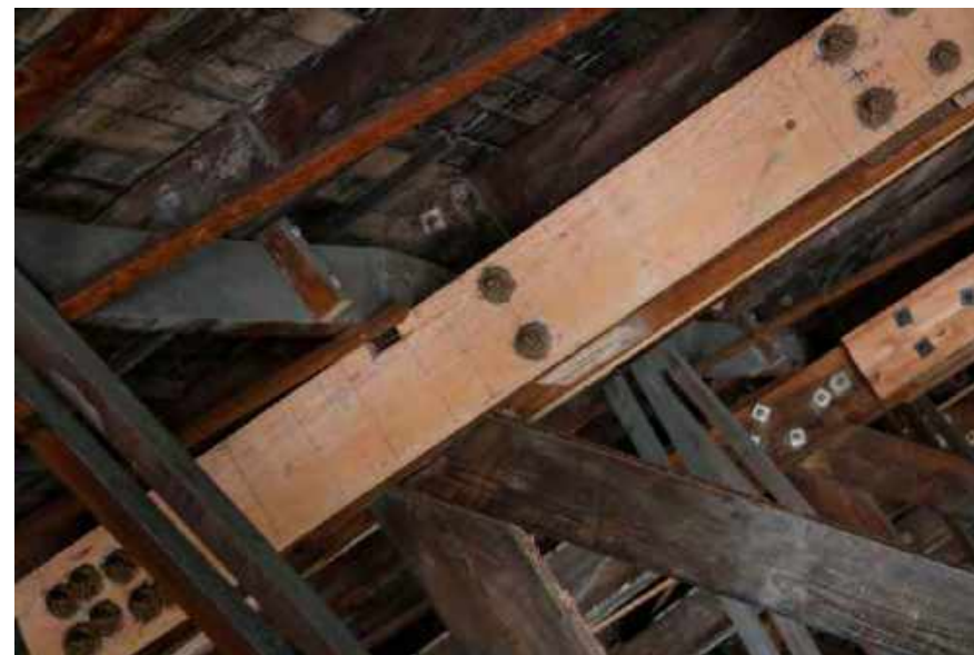
Chord sister repair installed prior to exoskeletons
