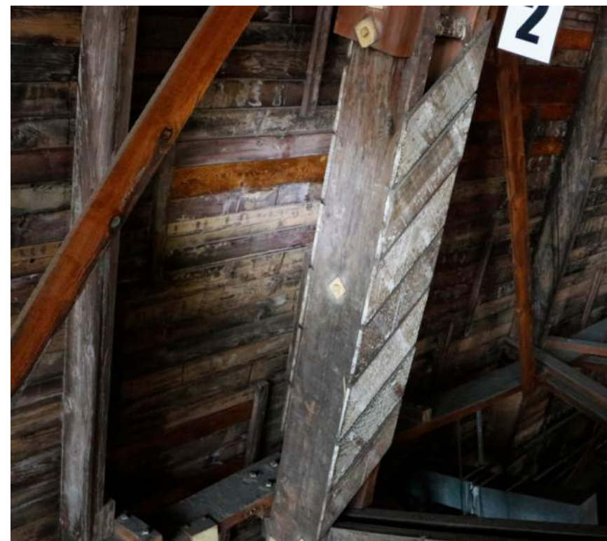
Typical chord member with battens
