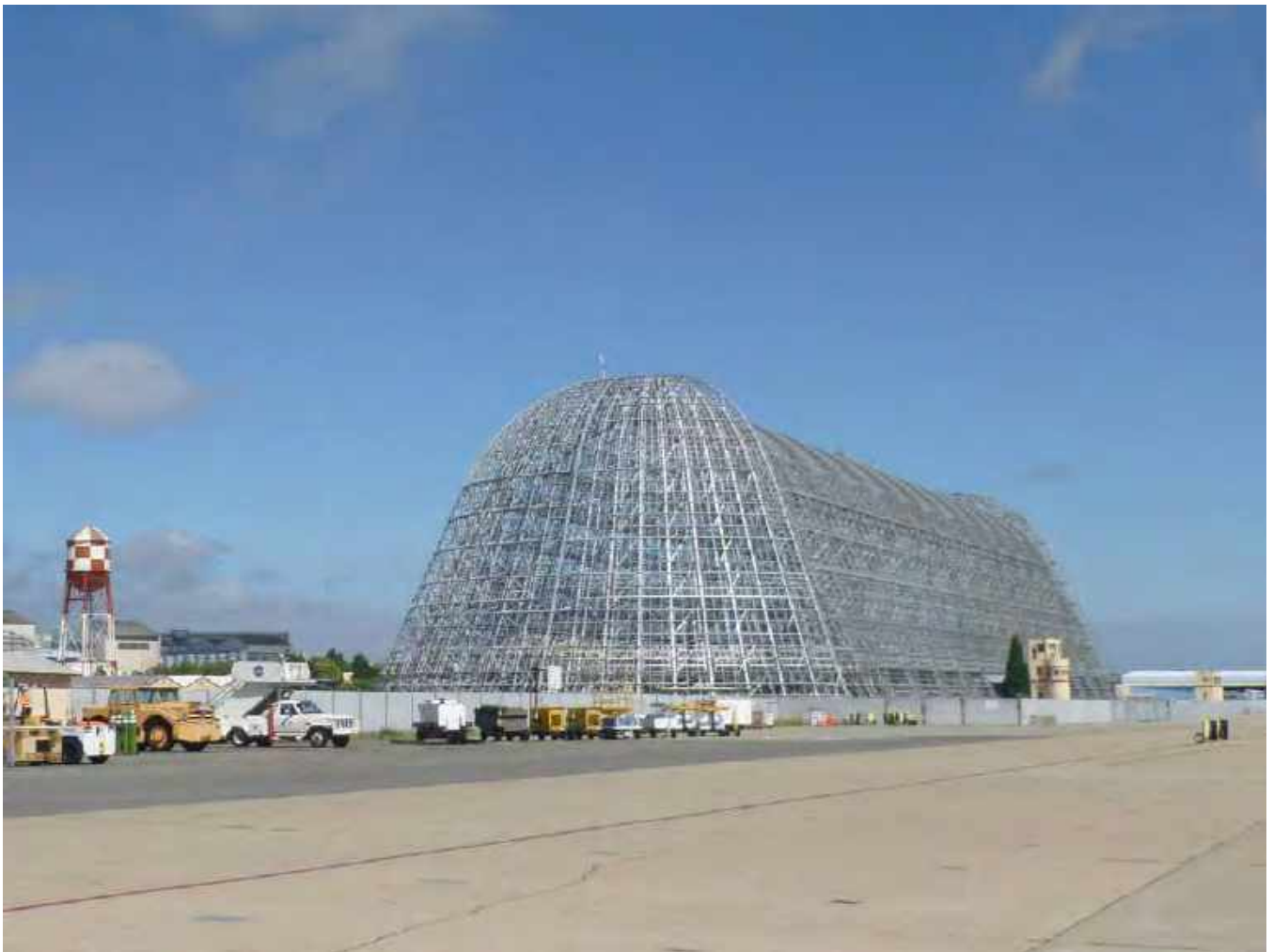
View of Hangar 1 looking northwest (Source: AECOM 2013)
