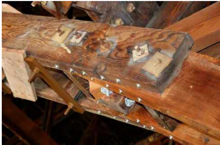
Preemptive screw and clamp strengthening on undamaged chord at node K
