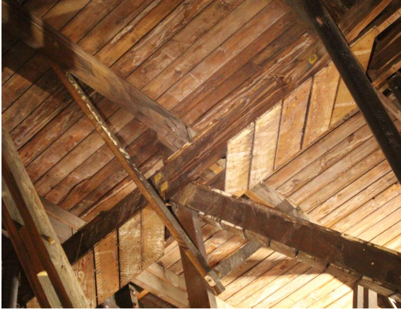
Typical vertical web member with added knee-braces
