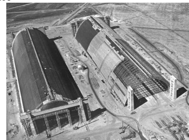
Hangars 2&3 under construction -US Navy Historic Photos
