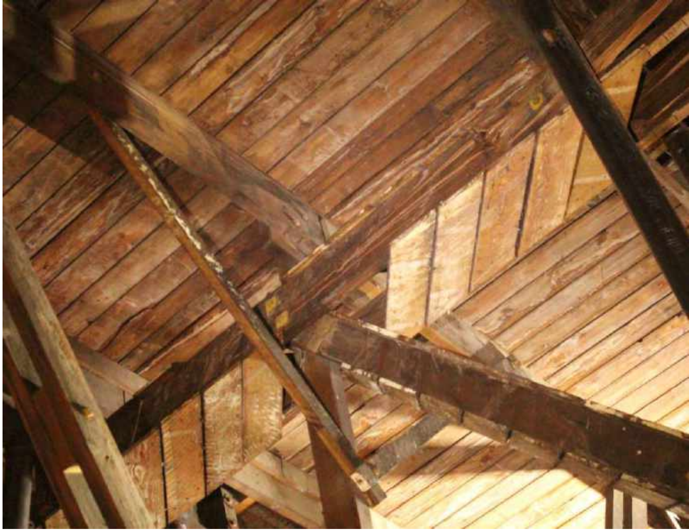
Typical vertical web member with added knee-braces
