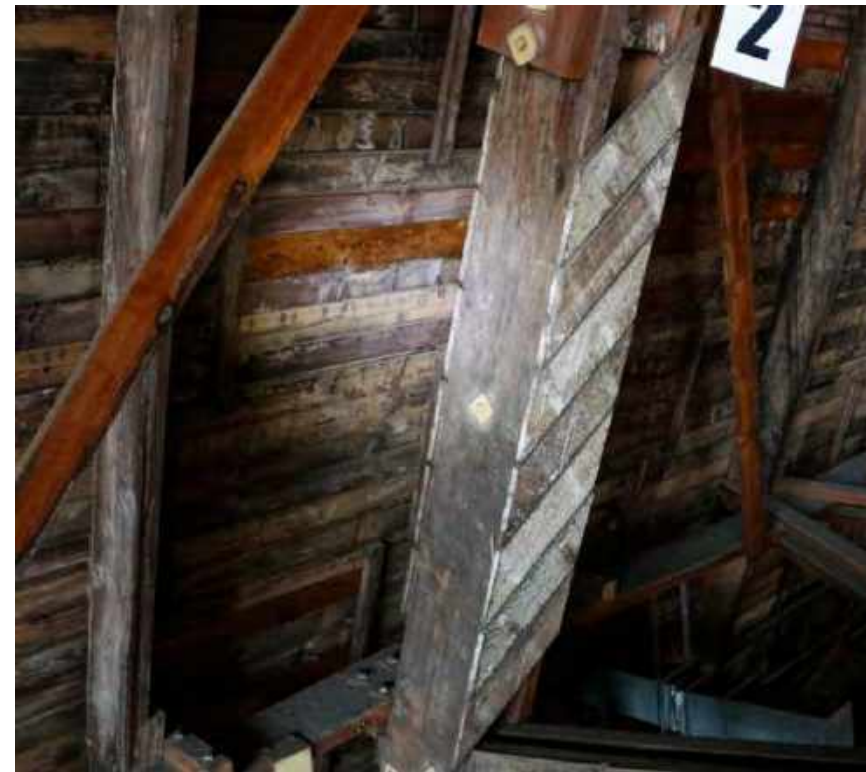
Typical chord member with battens
