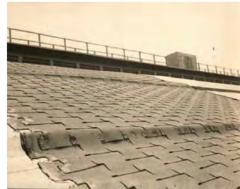
Asphalt shingles documented in 1954 -Seabees Historic Photos
