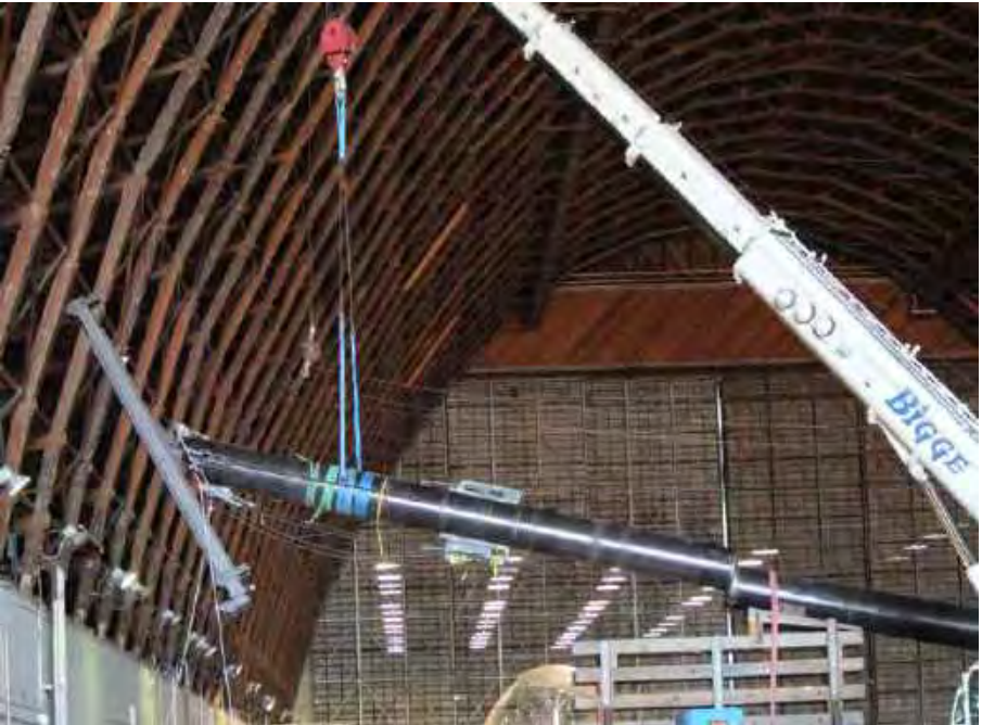
Hoisting of temporary shore segment
