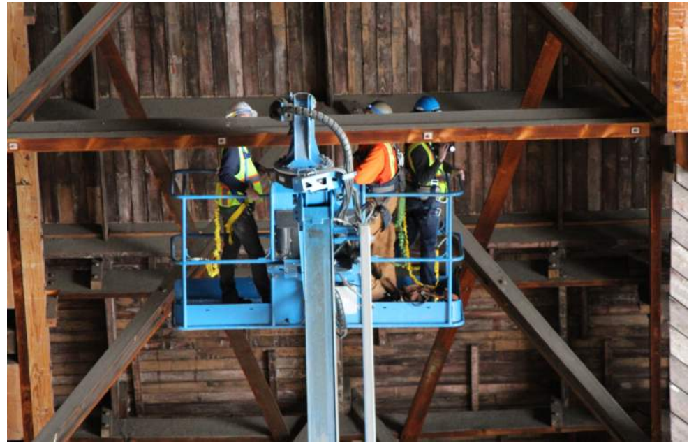
KPFF condition assessment crew
