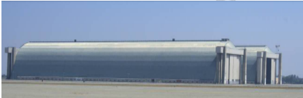
Figure 2. 2013 Hangar 2 (nearest hangar) and Hangar 3.
