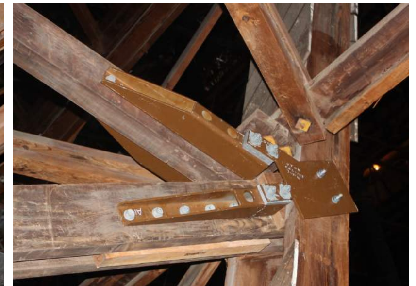
Typical connection strengthening bracket
