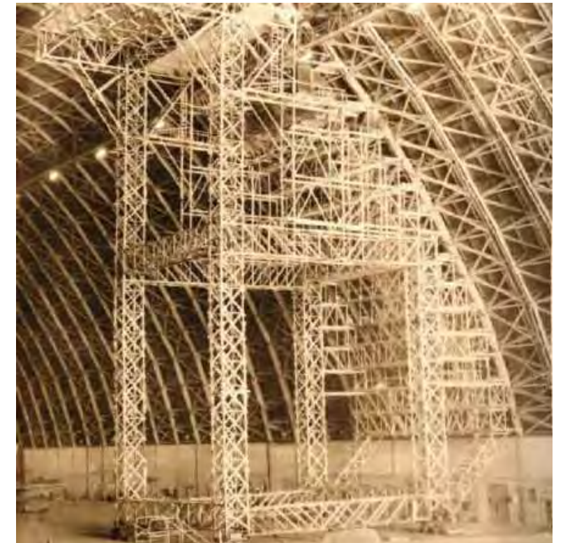
Rolling scaffold used to install battens - Seabees Historic Photos
