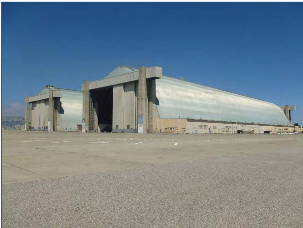
Photograph 4: South and east elevation of Hangar 3 with Hangar 2 in the background.
