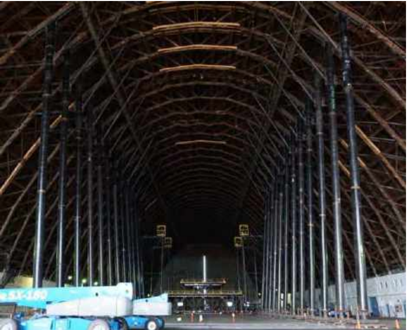
Temporary shores after installation
