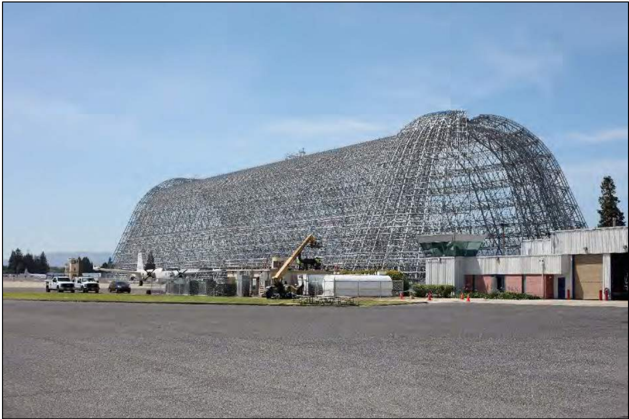
Photograph 3: North and east elevations of Hangar 1, looking south.
