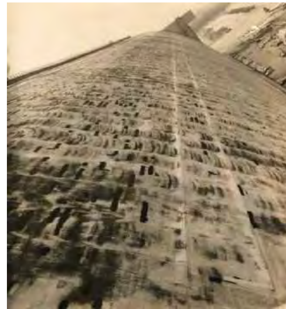
Original roofing system -Seabees Historic Photos
