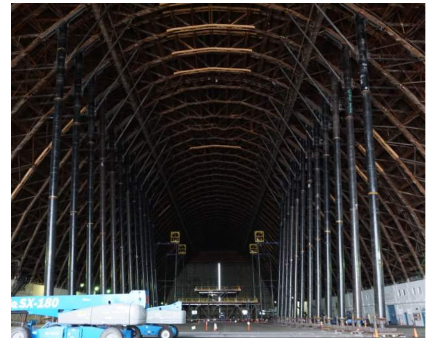
Temporary shores after installation
