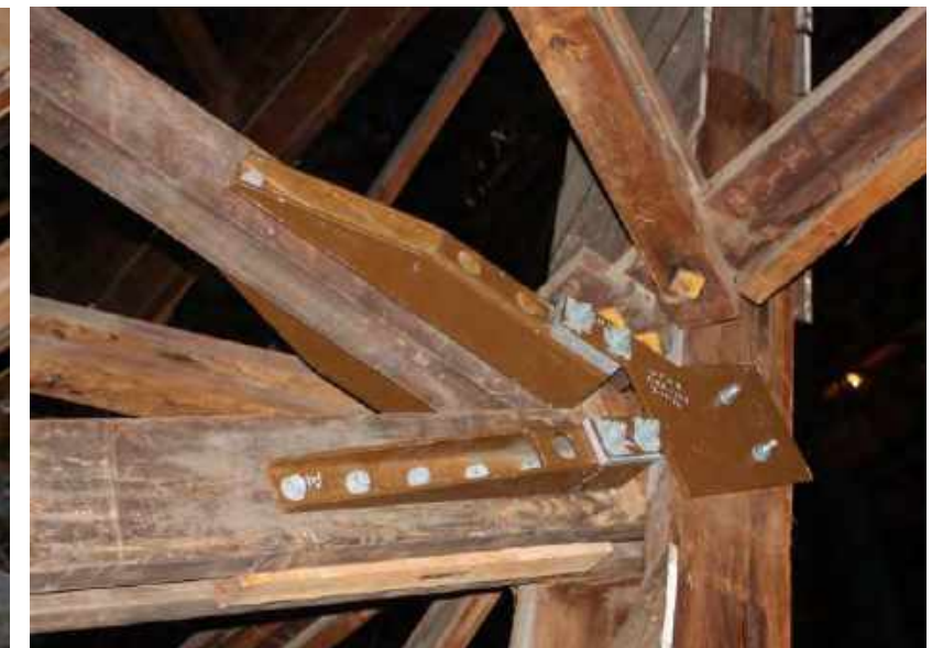
Typical connection strengthening bracket
