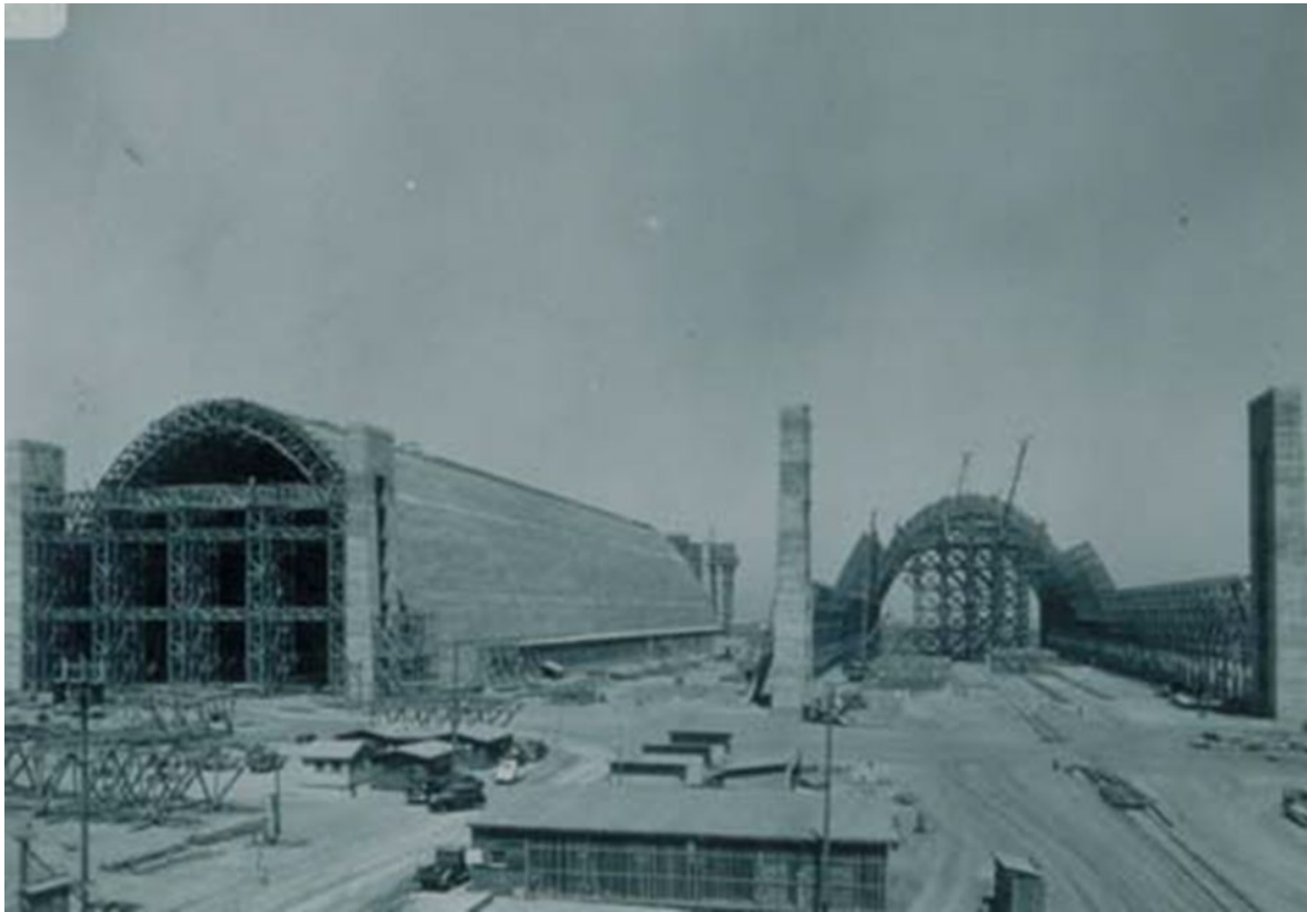
Photo 1: Hangars 2 and 3 Under Construction, 1943
