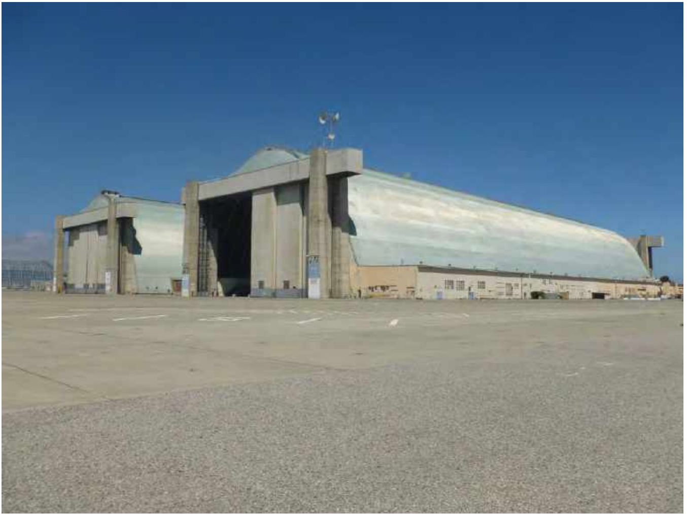
View of Hangars 2 and 3 looking northwest ( Source: AECOM 2013 )
